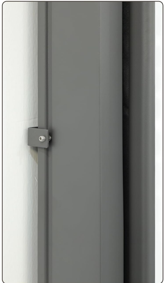
Image: Detailed view of how the side awning leg tube is clamped with a metal bracket and anchored to a wall.
