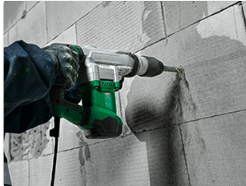
Drilling into a concrete wall.
