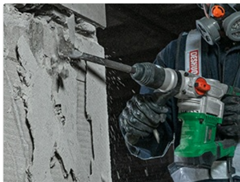
Chipping concrete with the hammer function.
