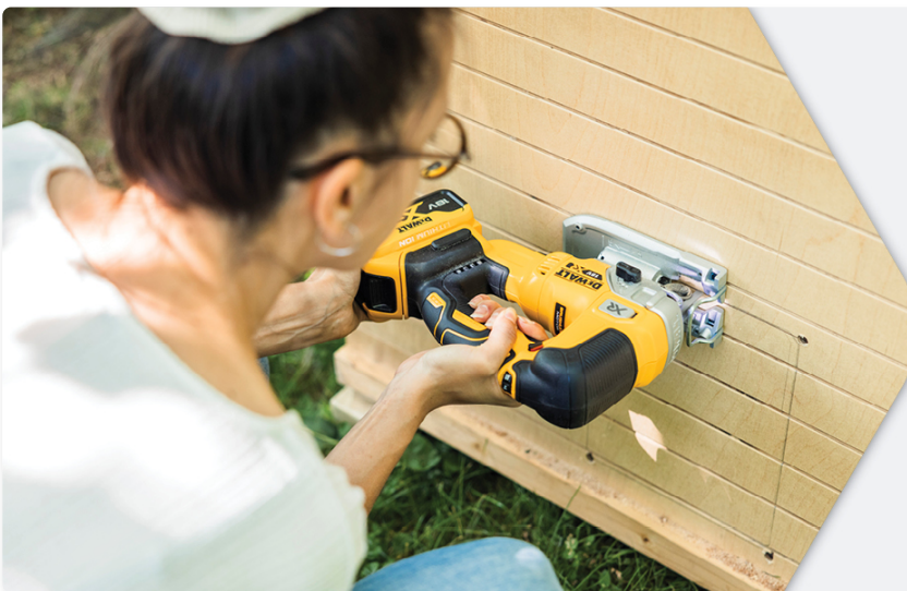
Image 3.2: Preparing the opening for the door using a template ensures a perfect fit.
