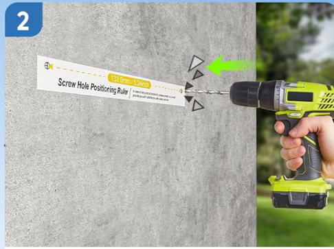
Drill marked holes
