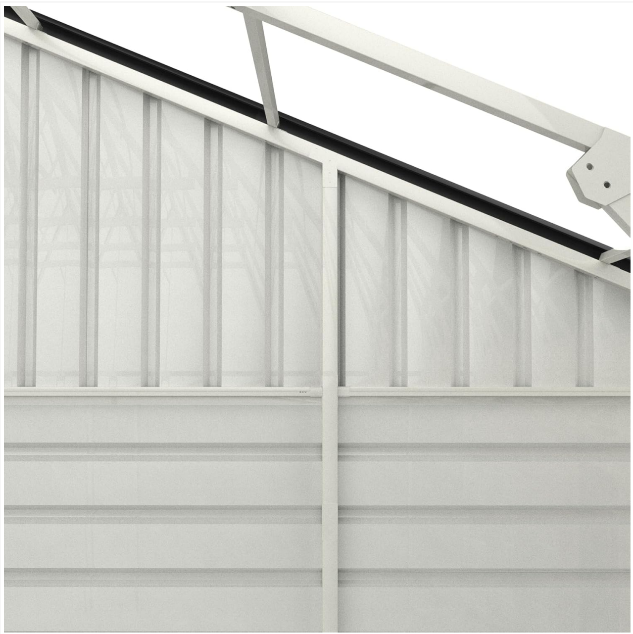
Figure 8: Interior wall and frame detail, showing the corrugated metal sheeting.
