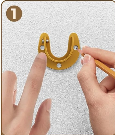
1 Mark the bracket hole positions
