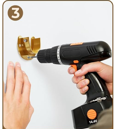
3 Secure the brackets with screws
