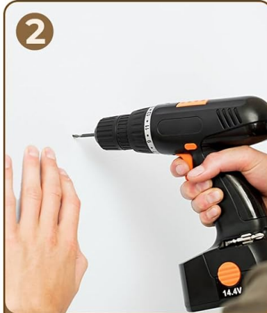
2 Drill holes and insert wall anchors
