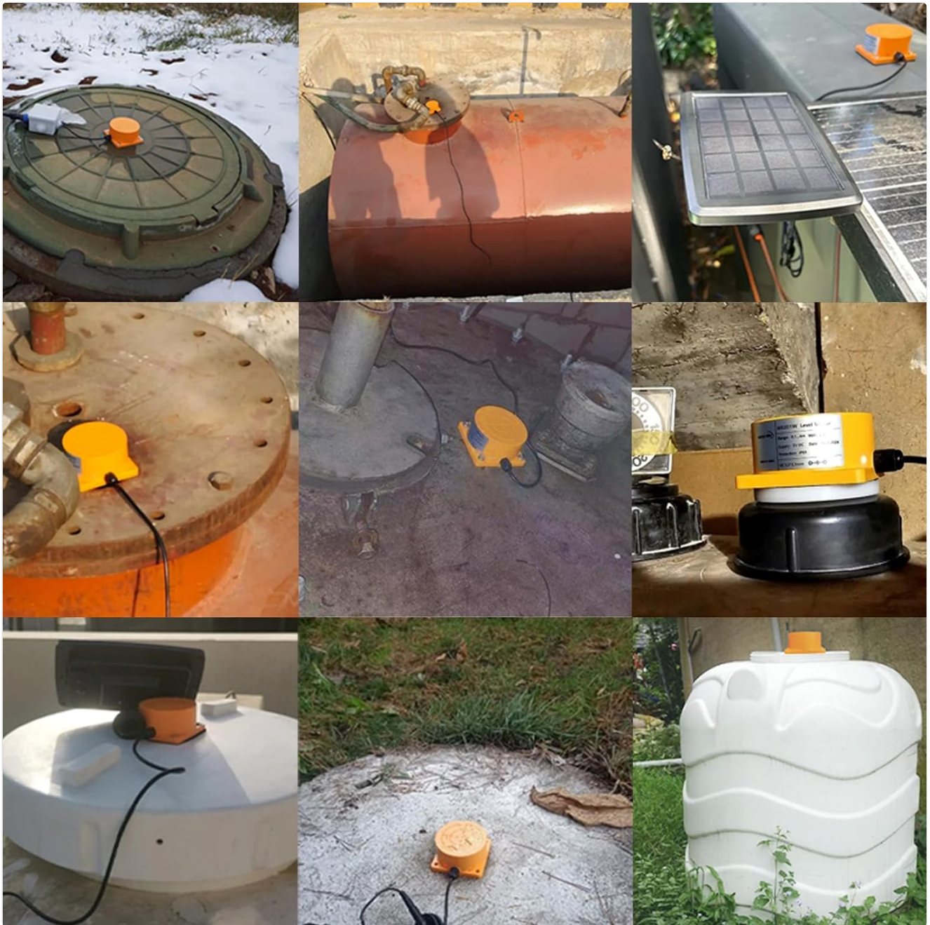
Figure 6.2: Examples of Sensor Installation on Various Tanks.
