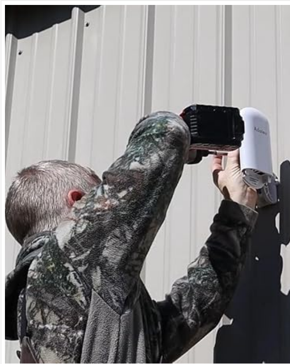
Image 5.1: Video transmission setup with CPE661 bridges.
