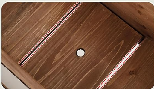
Gaps Between the Plates
