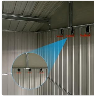
Image 6.1: An example of hooks installed on the interior wall of the shed, demonstrating how the reinforced steel columns can be used for organized storage of tools and equipment.
