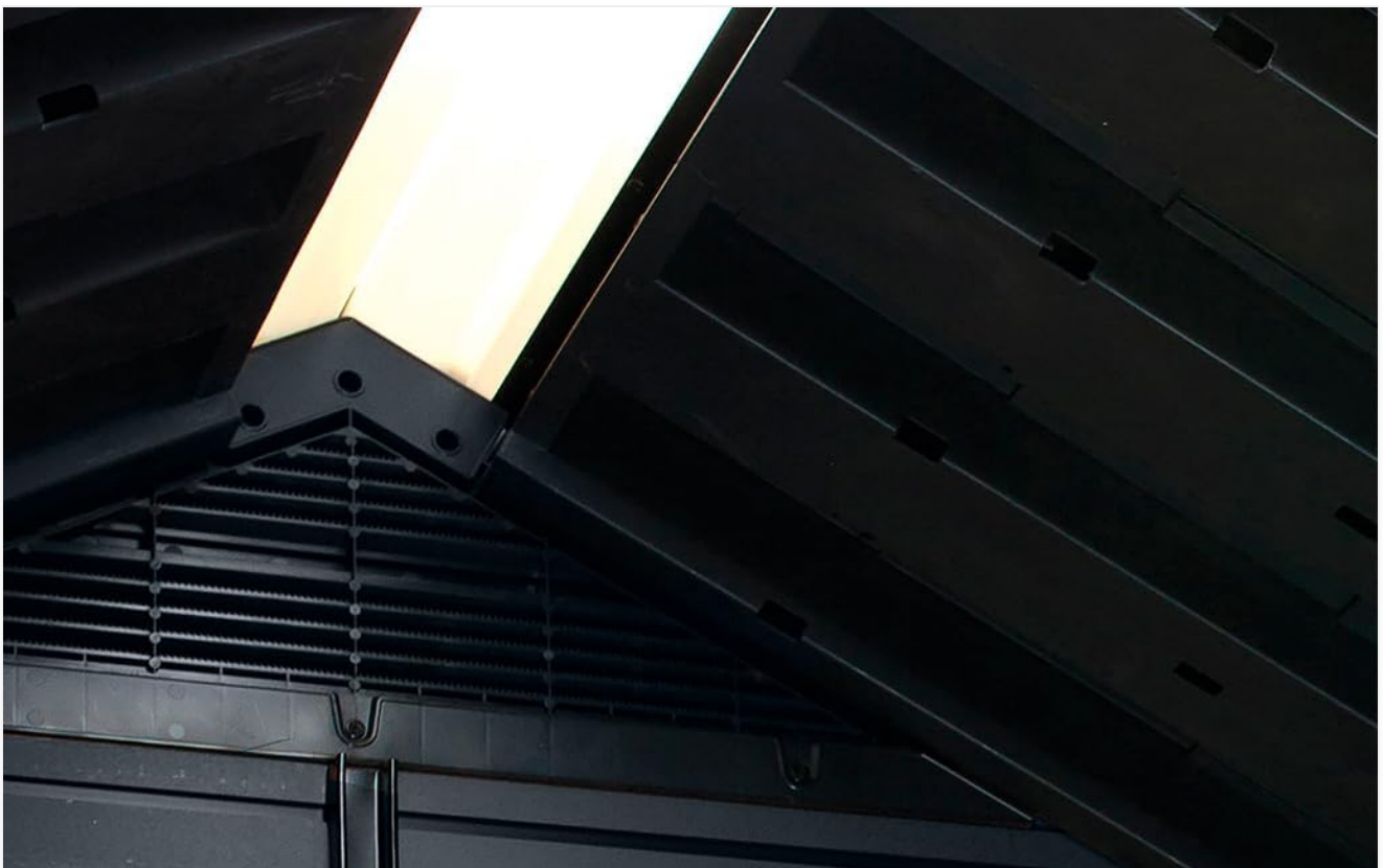
Image 5.2: Interior view highlighting the continuous skylight and integrated ventilation system for natural light and air circulation.
