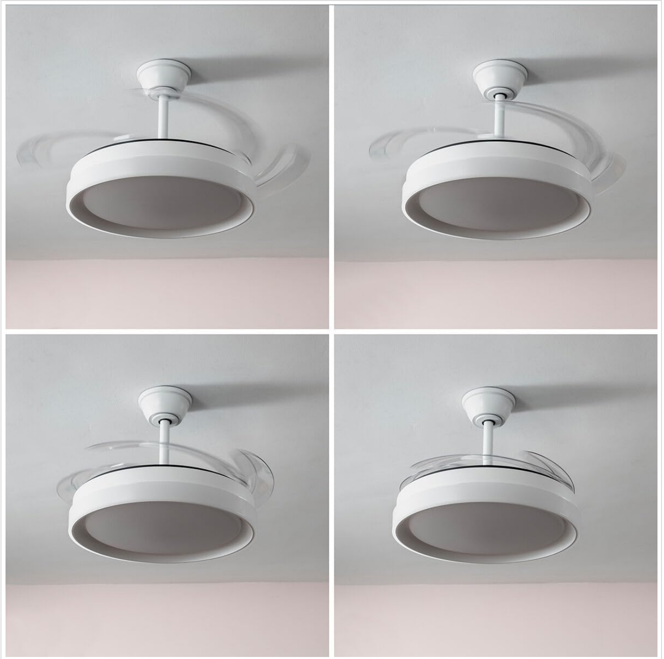
Image: A four-panel sequence demonstrating the fan blades transitioning from extended to fully retracted positions.
