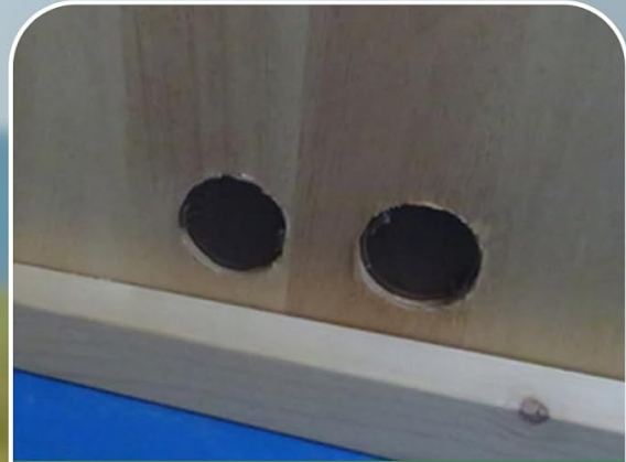
Dual Inlets for Wires & Pipes
