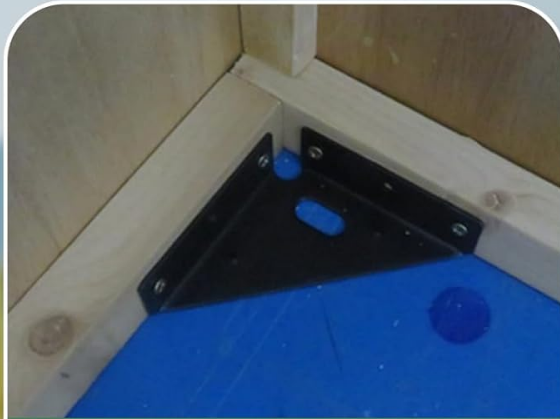
Triangular Reinforcement Bracket
