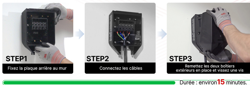
Image 3.2: Simplified installation process for the ELECQ Wallbox.
