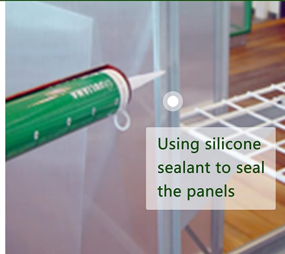
Image: Recommendations for increasing the greenhouse's wind rating, showing how to bolt the greenhouse to the ground and use silicone sealant to seal panels.
