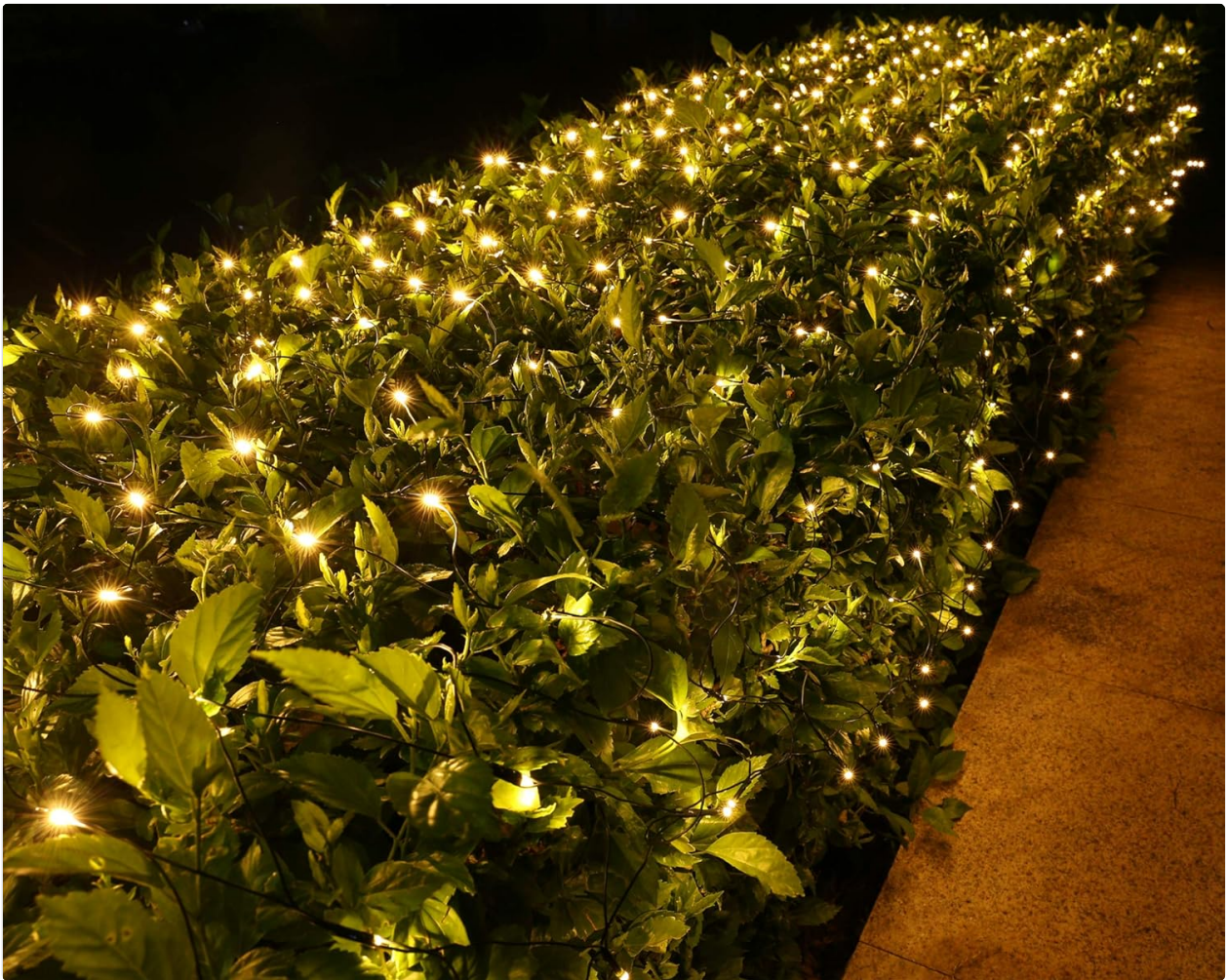
Image 1.1: Joomer Christmas Net Lights installed on a bush.
