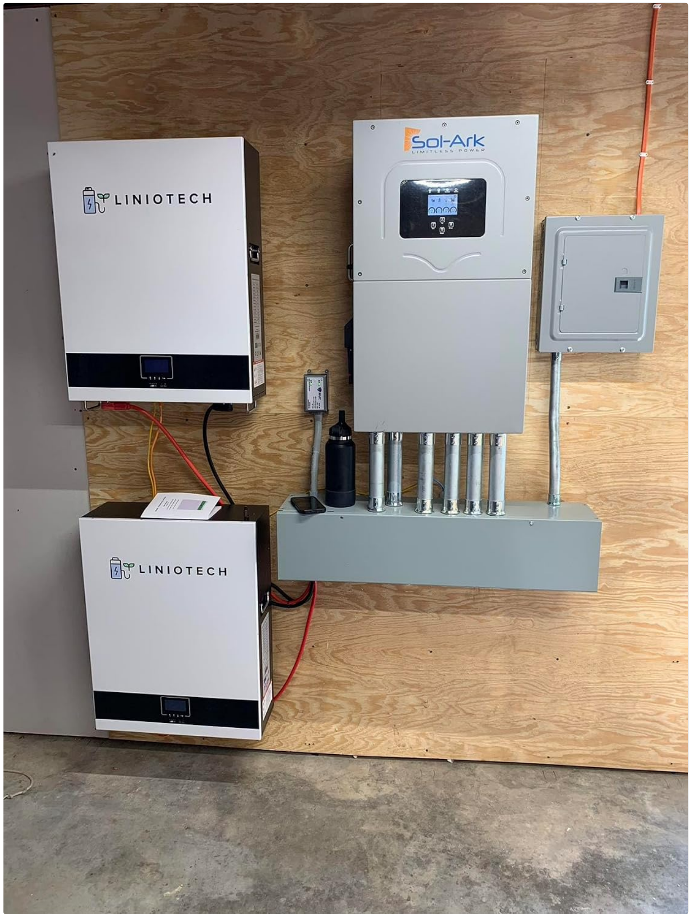
Figure 4.2: Example installation of the Sol-Ark 15K inverter alongside two Liniotech battery units, demonstrating typical wiring and conduit setup.
