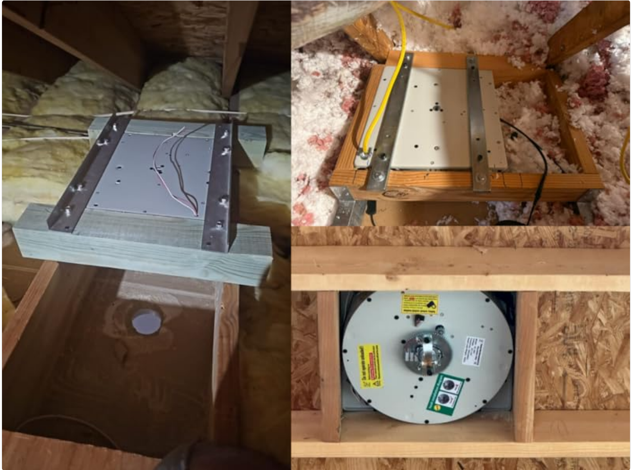
Figure 4.3: Illustration of hidden installation (left) where the lift is concealed within the ceiling, and surface installation (right) where a decorative cover is used.
