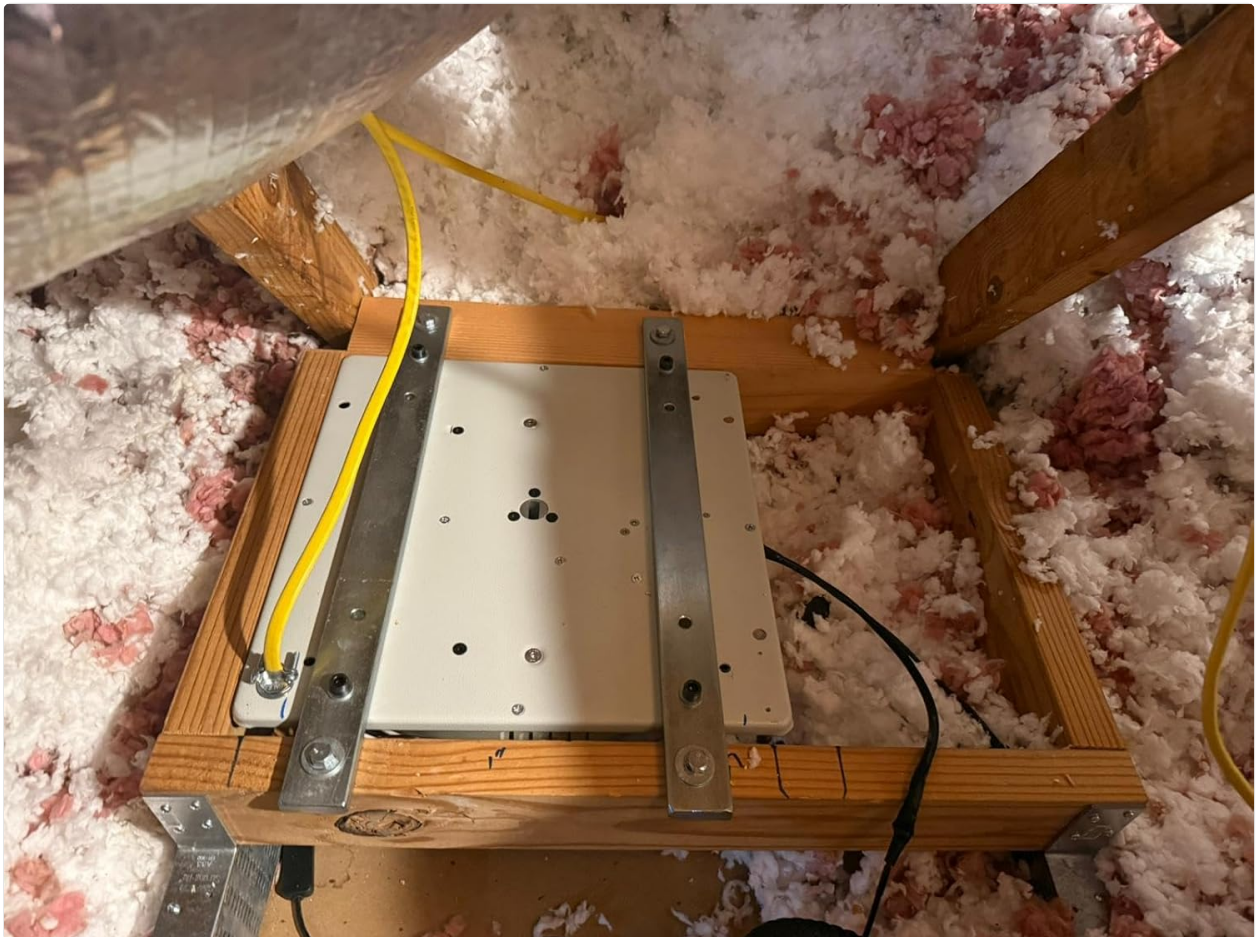
Figure 4.1: Chandelier lift system mounted within attic joists, demonstrating the use of wooden blocks and metal brackets for secure installation.
