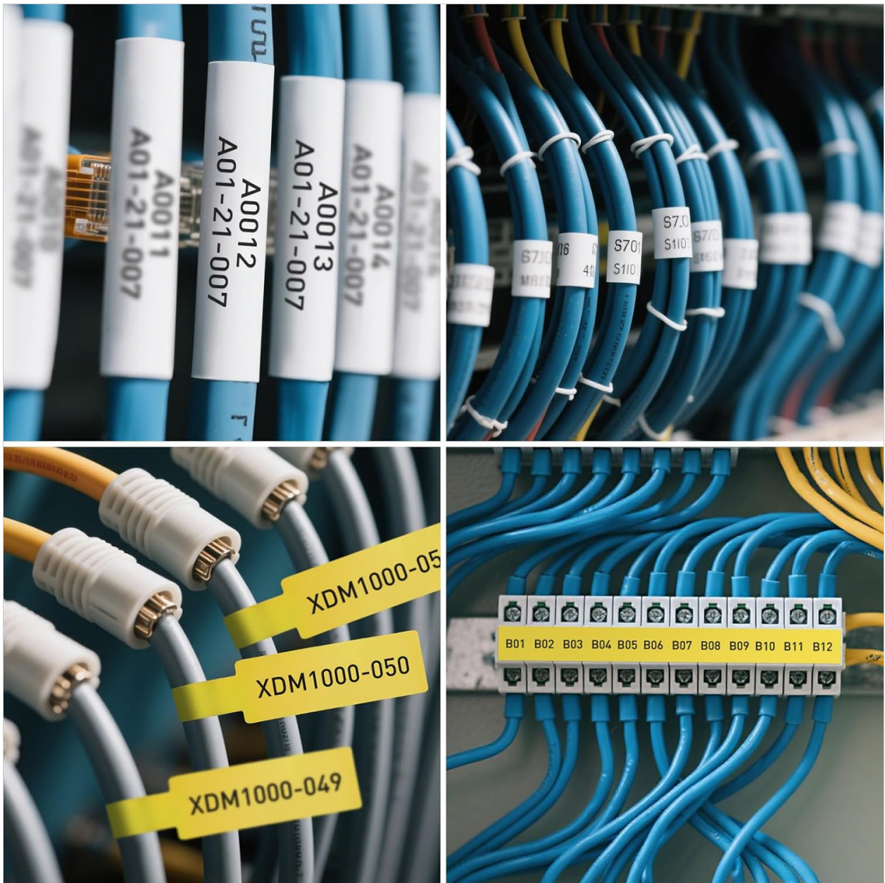
Figure 4: Examples of SUPVAN wrap-around labels on various cables. This image collage shows multiple applications of the wrap-around labels on different types of cables, including network cables, power cords, and electrical wiring, demonstrating their versatility.
