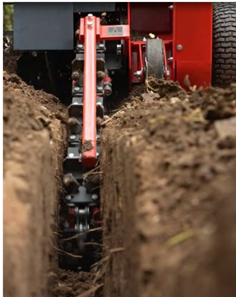
Figure 5.1: The trencher efficiently digging a trench in soil.
