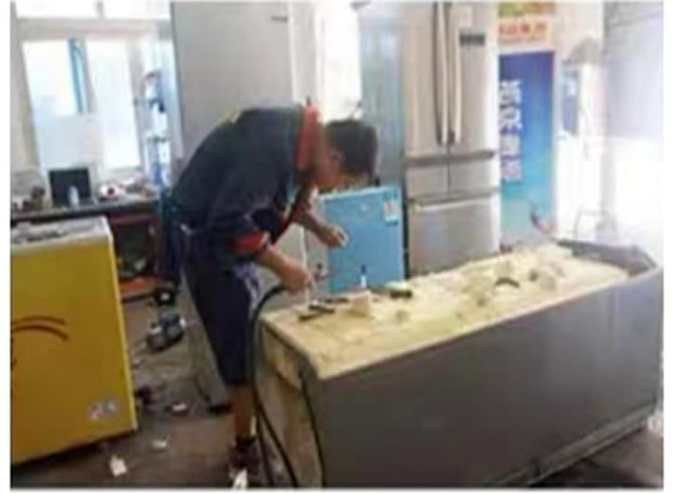
Refrigerators Cold Insulation
