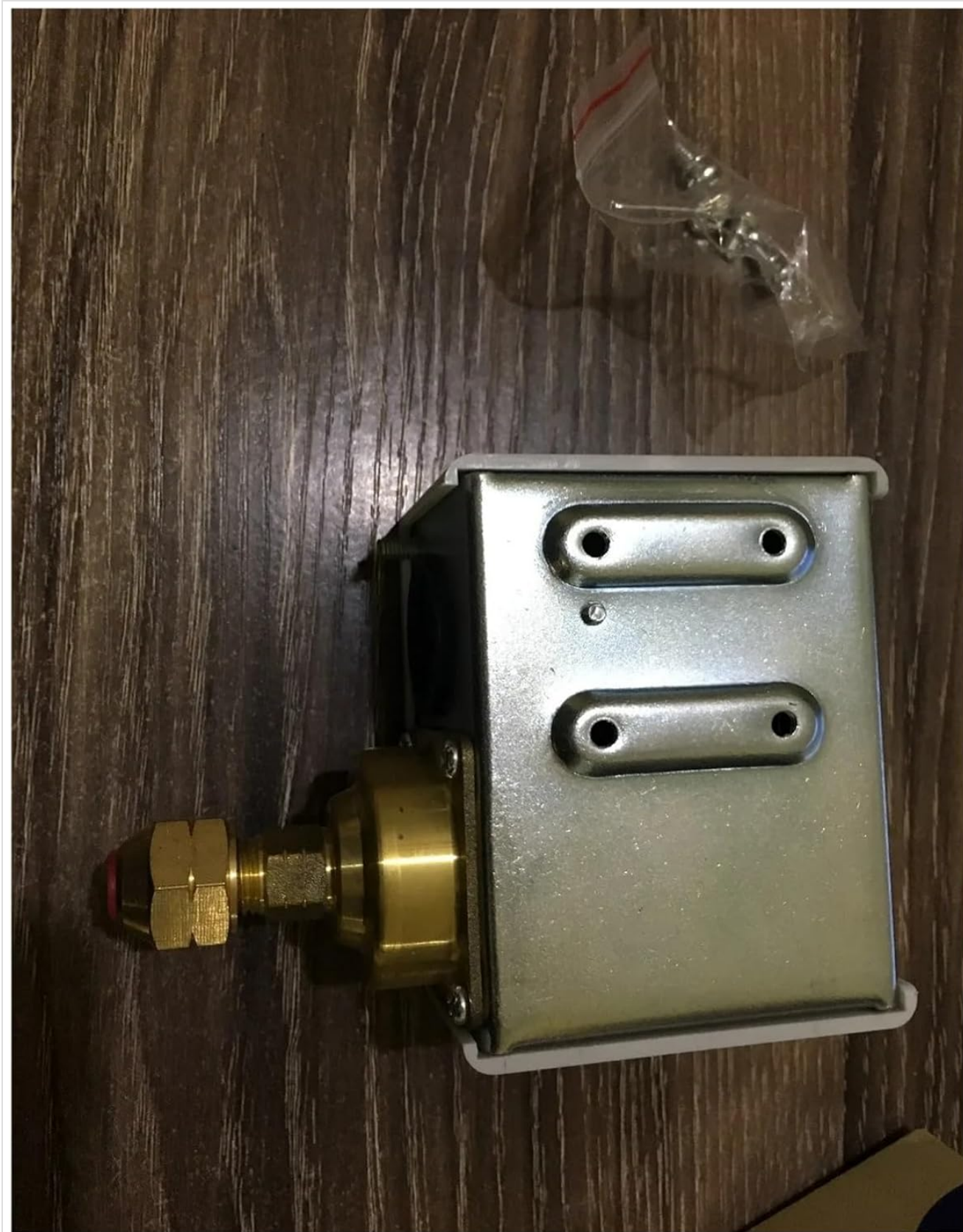
Figure 2: Bottom view of the PYKFVTGL Jc-230 Pressure Switch Controller, revealing the metal casing and mounting holes, with the brass pressure fitting visible.
