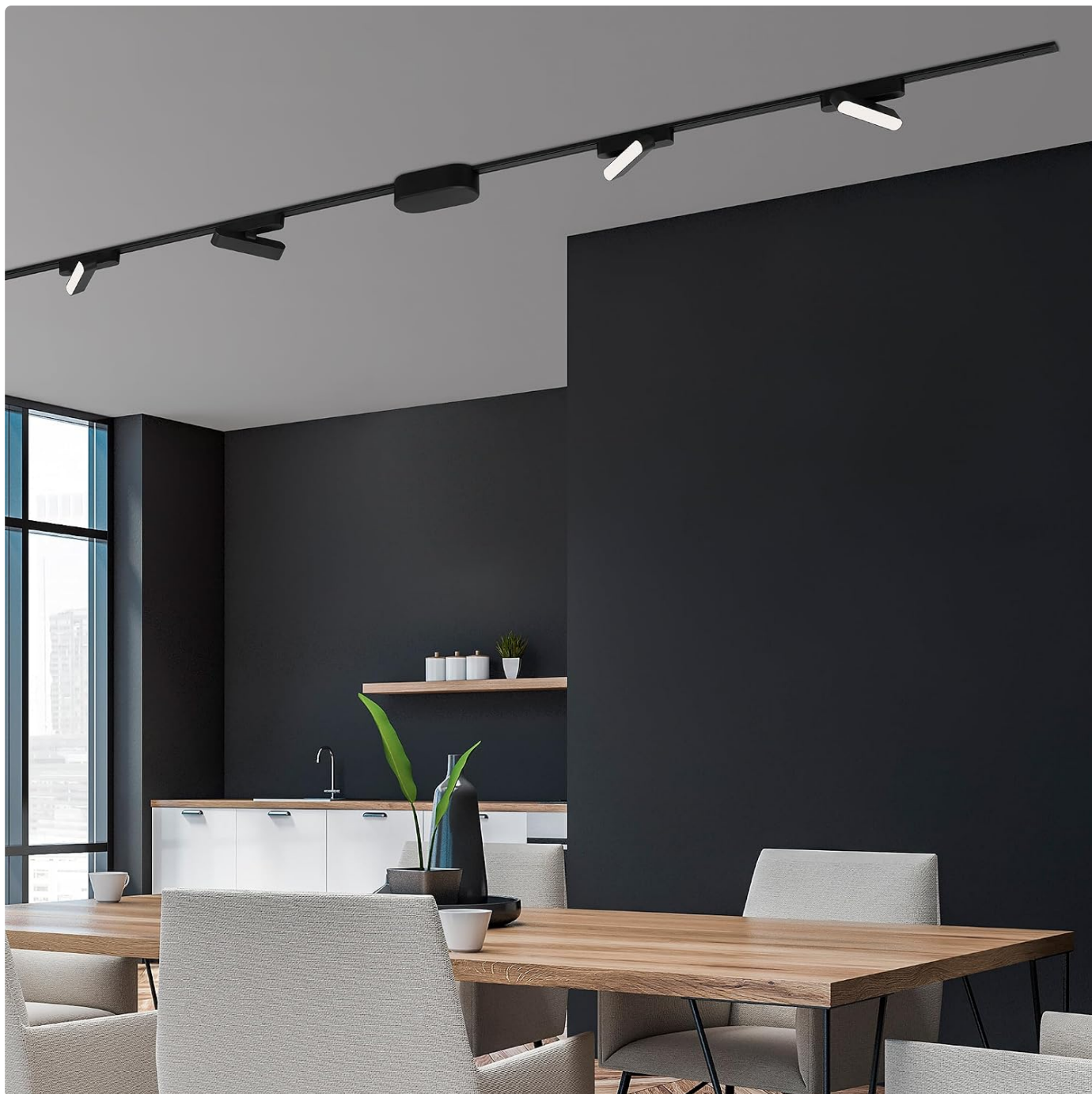
Image: An example of the tracklight system installed in a dining area, providing clear and defined lighting.
