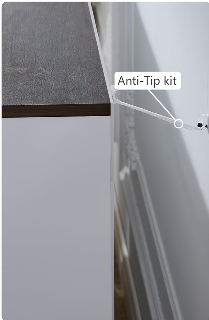
Image 2.1: Illustration of the anti-tip kit installation and the importance of securing the dresser.
