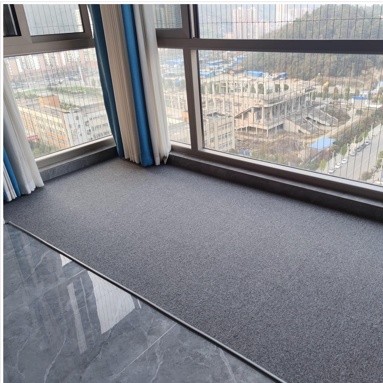
Image: A wide shot of a room with the carpet edge trim successfully installed, providing a neat finish to the carpeted area.
