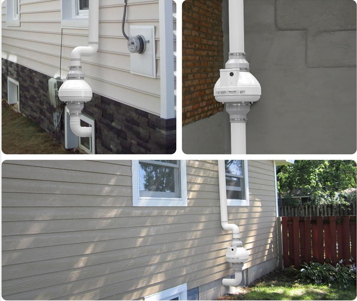
Image 3.4: This image displays examples of the BaseAire RadonEx 15F fan installed outdoors, demonstrating its weather resistance and suitability for external mounting on a building's exterior.
