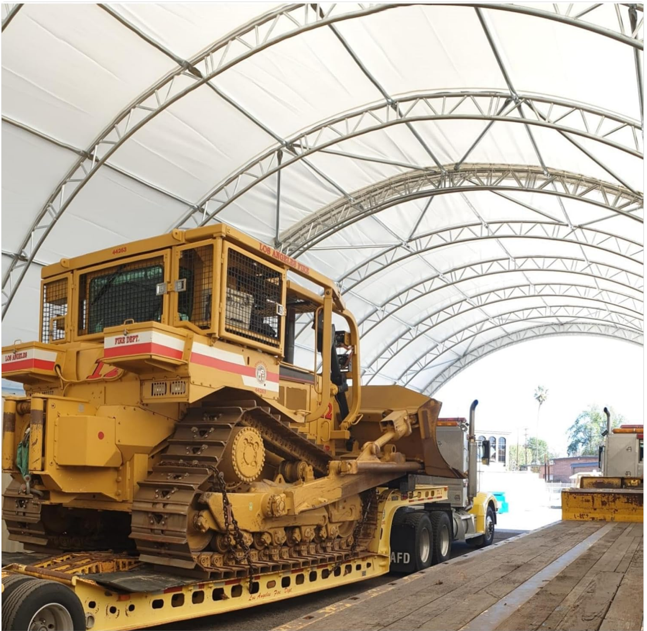
Figure 3: Multiple truss sections forming the canopy structure.
