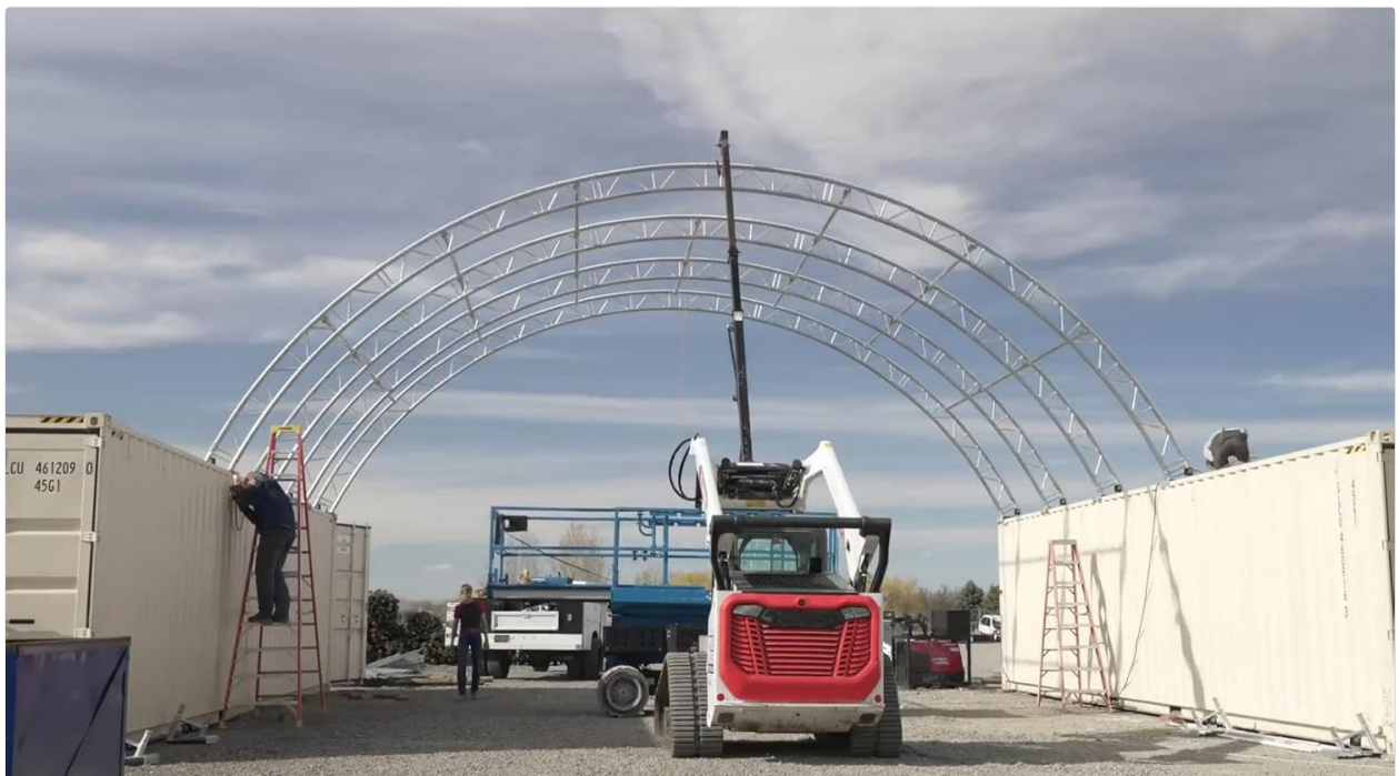
Figure 2: Lifting and positioning a truss section during assembly.
