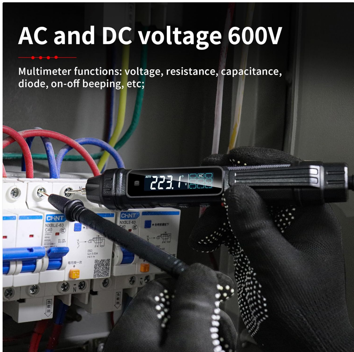
Figure 5.1: Measuring AC voltage in an electrical panel.
