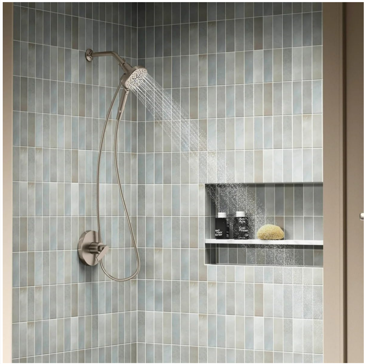
Figure 2: The Kohler Tellin Handshower installed, showing the magnetic dock and flexible hose.
