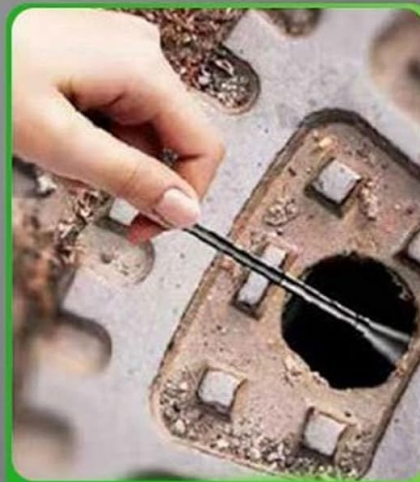
Clogged Pipes Inspection
