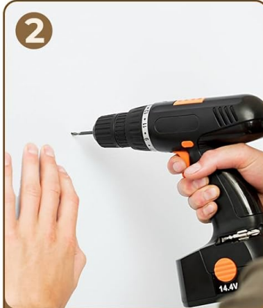
2 Drill holes and insert wall anchors
