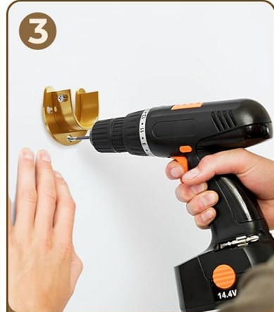
3 Secure the brackets with screws
