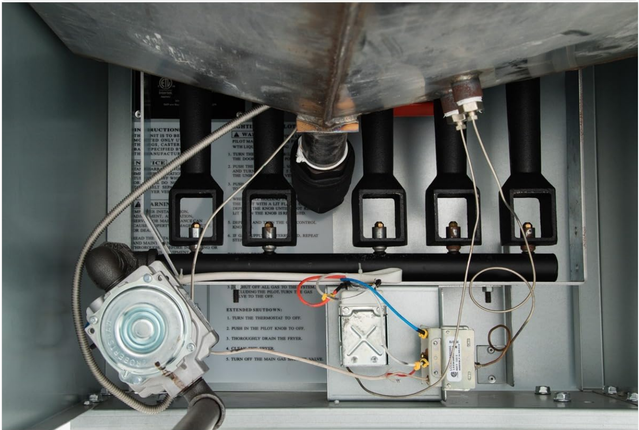
Image 3.1: Interior view showing the gas valve and burner tubes. This area requires professional installation and maintenance.
