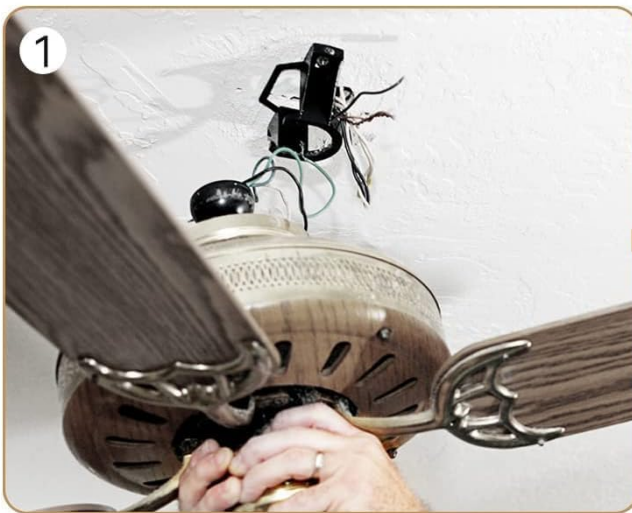
1 Disconnect the ceiling fan wiring
