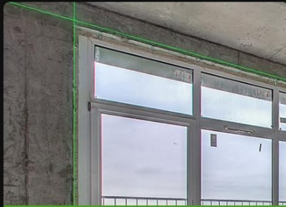
Door and Window Installation
