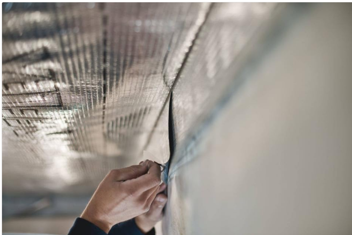
Figure 2: Close-up view of hands applying FireMaster FastWrap XL to a duct, demonstrating the process of securing the material and ensuring proper seam alignment.
