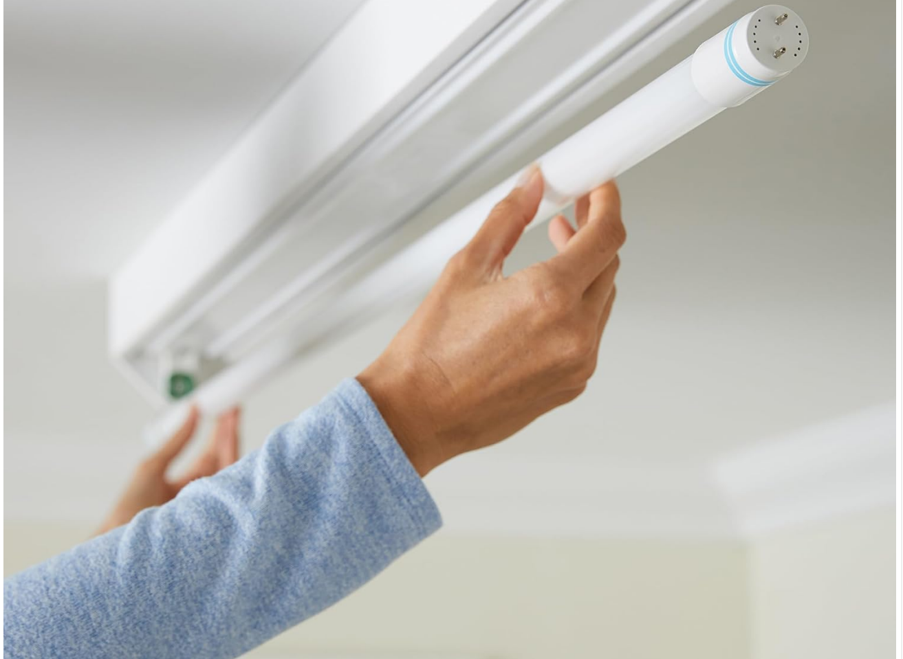
Figure 4: A close-up view of a Philips LED tube being installed into a ceiling fixture, emphasizing its compatibility with most electronic and magnetic ballasts.
