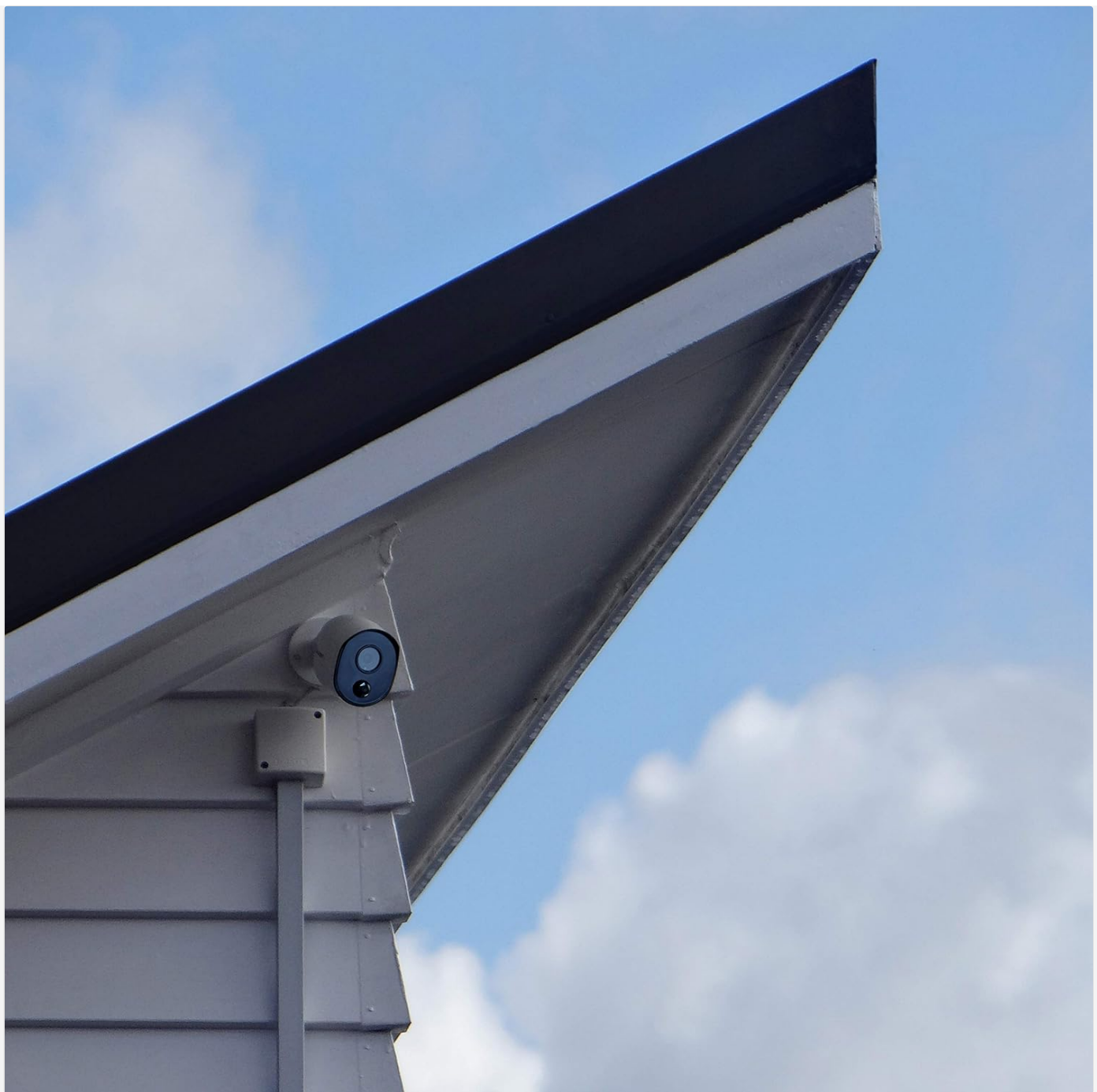
Image 3.2: Camera mounted on an exterior wall.
