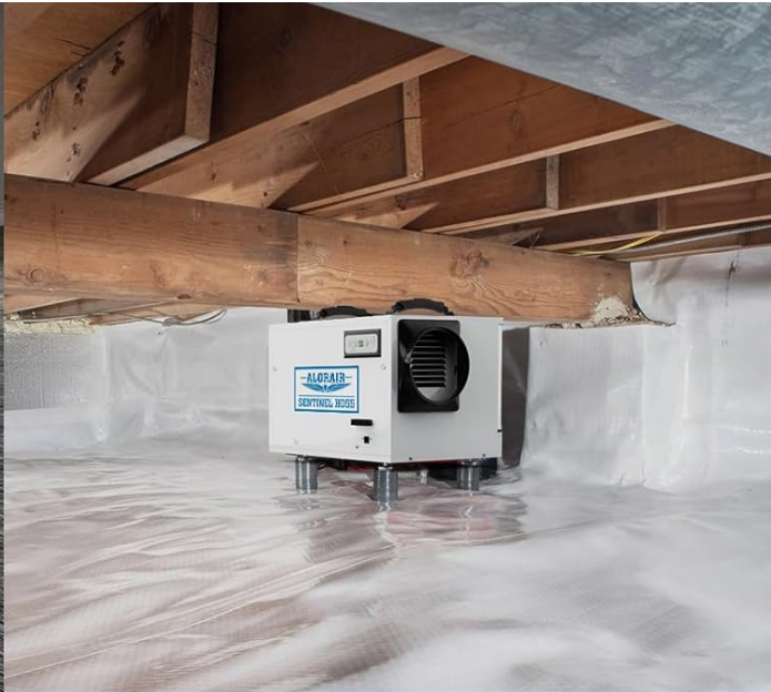
Crawl Space Dehumidifying
