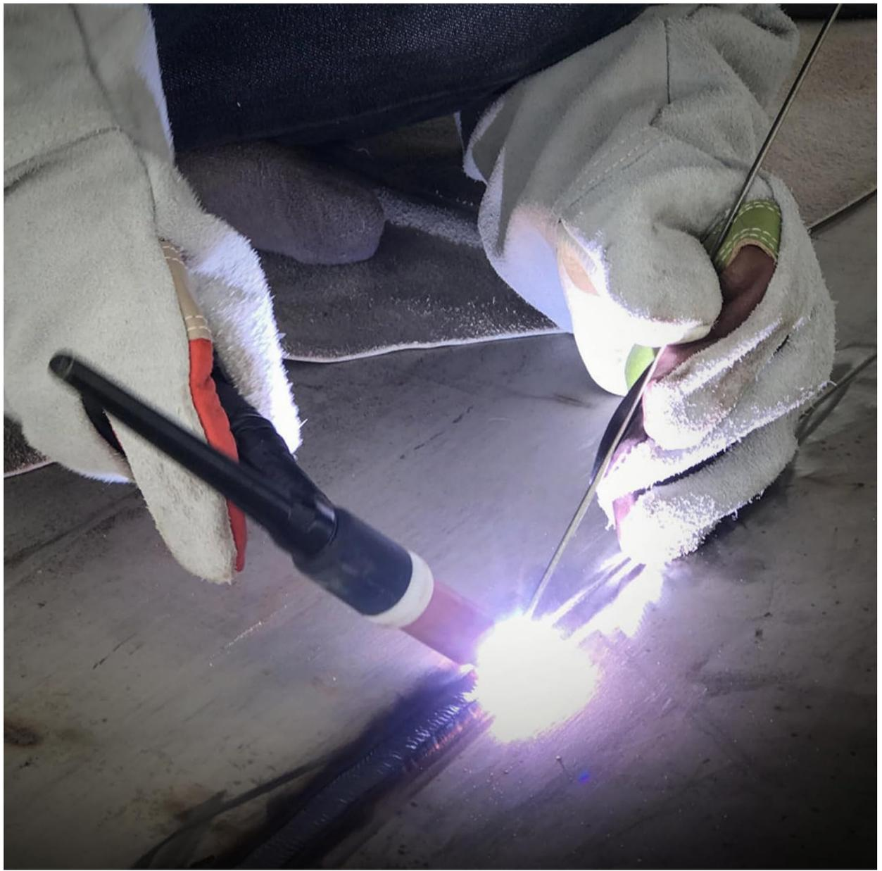
Figure 7: An operator performing Lift TIG welding.
