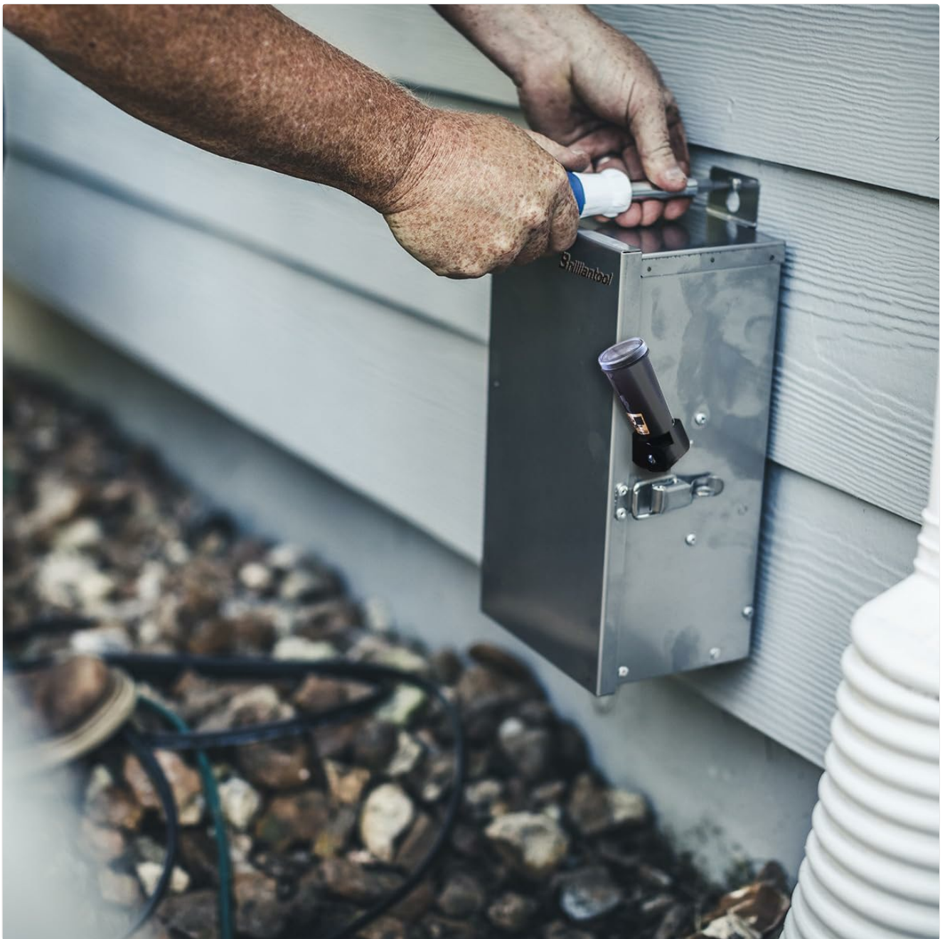
Image Description: This image depicts a person using a screwdriver to mount the Brilliantool low voltage transformer onto the exterior siding of a house. The transformer is positioned at a convenient height for installation.
