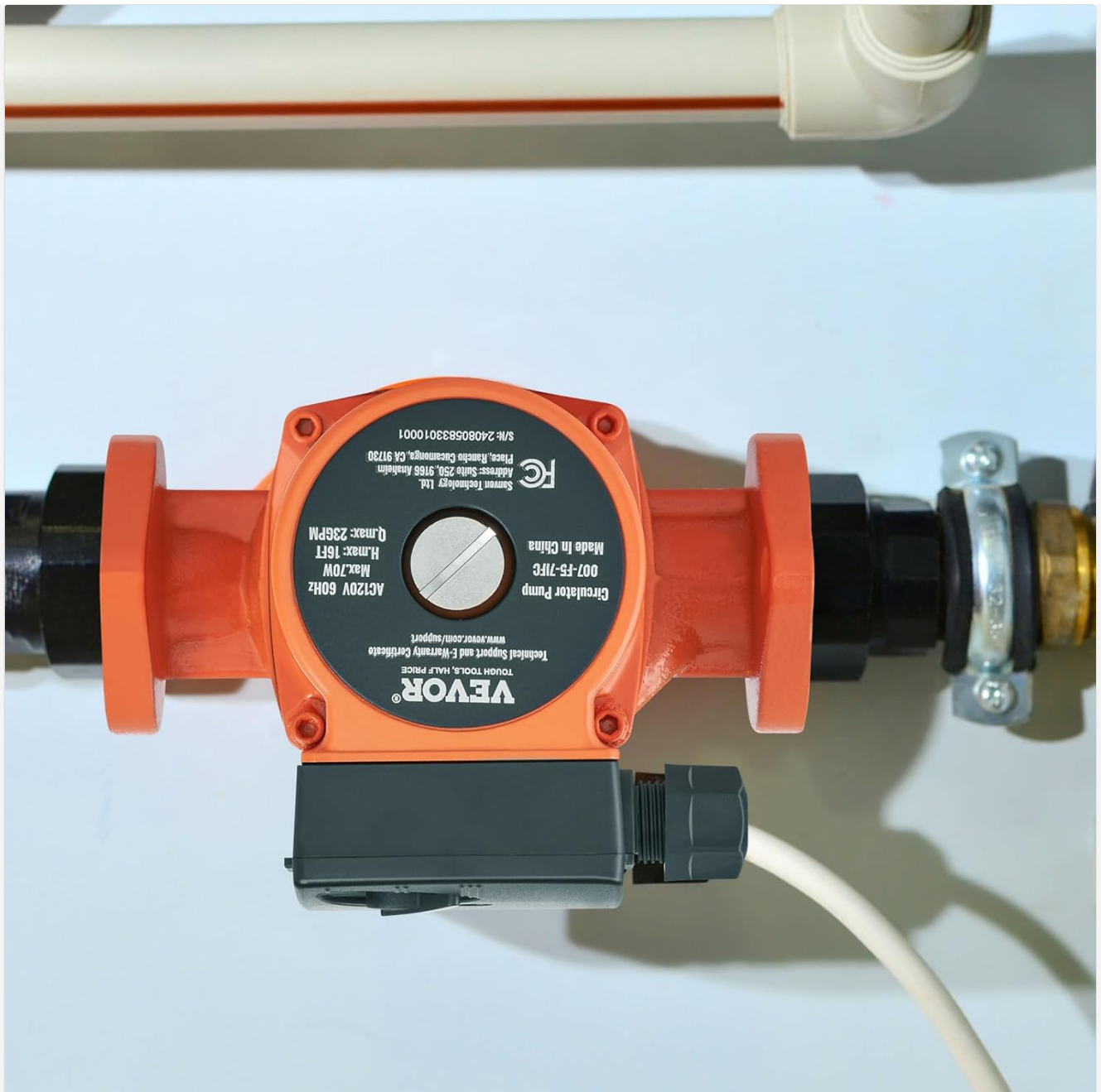
Figure 5: Example of the VEVOR 007-F5-7IFC Circulation Pump installed within a heating system.
