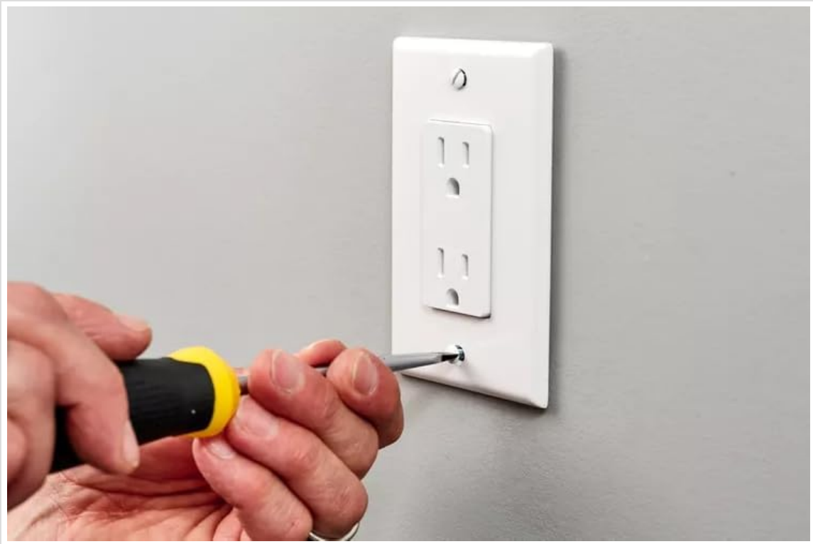
Figure 5.3: Attaching the faceplate to the installed wall outlet camera.
