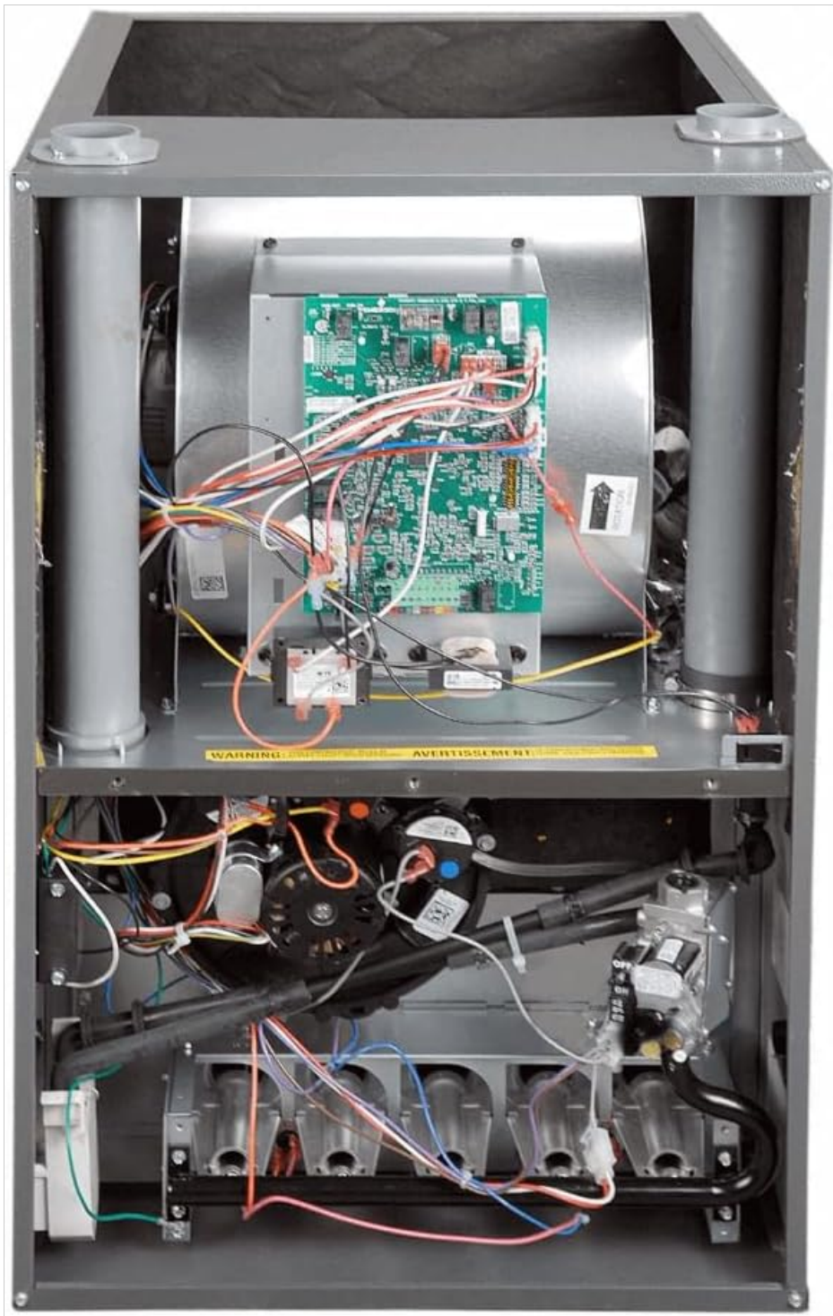
Figure 2: Internal view of the Goodman GD9S960403BN Gas Furnace. This image displays the complex wiring, circuit board, blower motor, and gas burner assembly within the unit, highlighting its sophisticated internal design.
