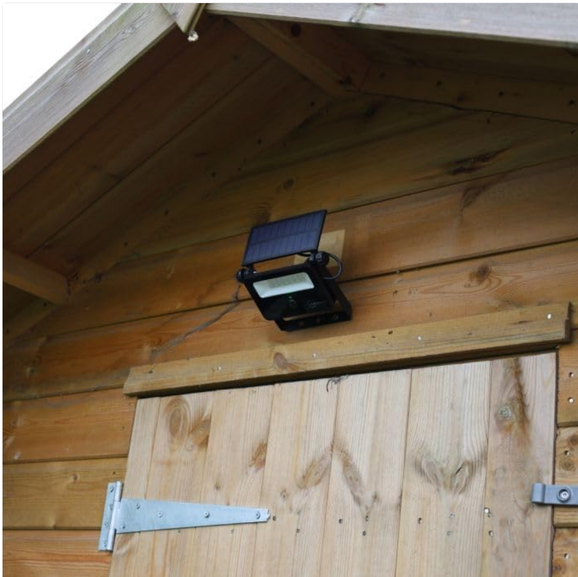
The Auraglow solar security spotlight is mounted on the wooden exterior of a shed, showcasing its suitability for wall or fence installation.
