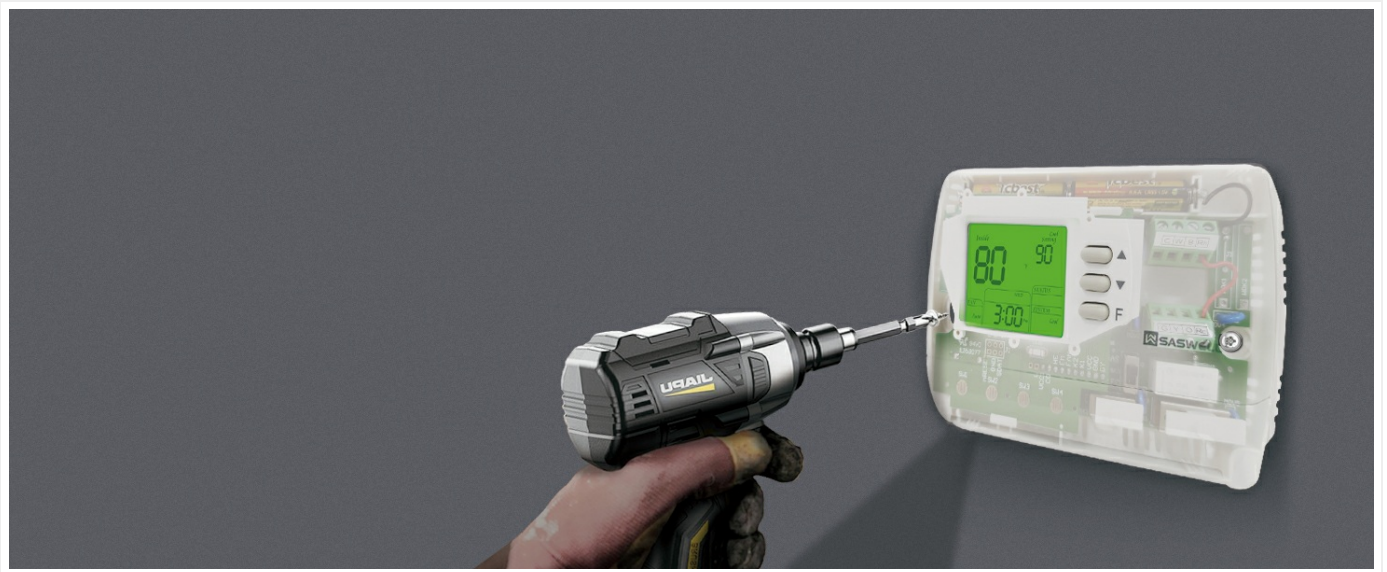
Figure 5.3: Illustration of thermostat installation.
