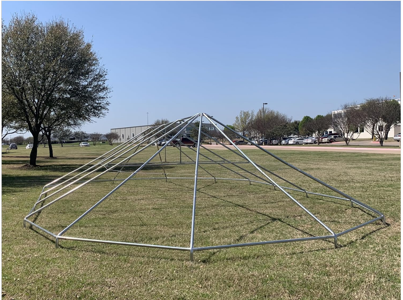
Image 3.2: The galvanized steel frame of the marquee tent during initial assembly, laid out on a grassy area.
