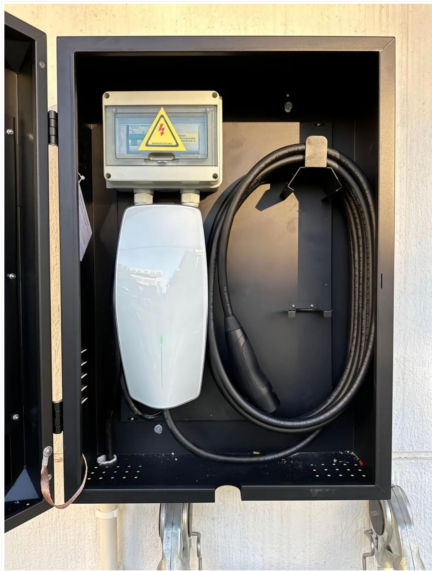
Figure 5.1: Example of an EV charger installed within the protective box.
