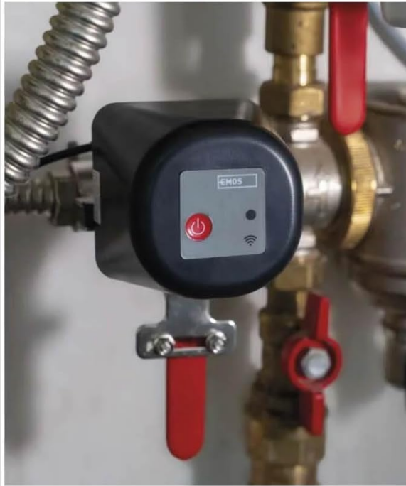
Figure 5.1: Installation on a Gas Valve
