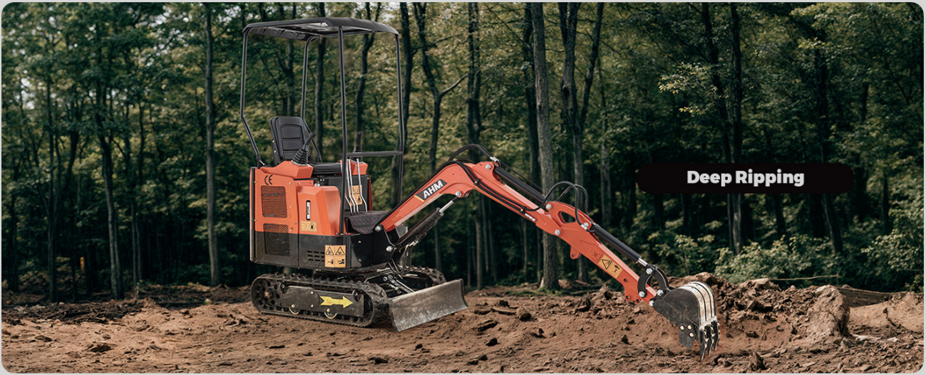
An example of the mini excavator being used for landscaping, demonstrating its ability to handle tasks in various outdoor environments.
