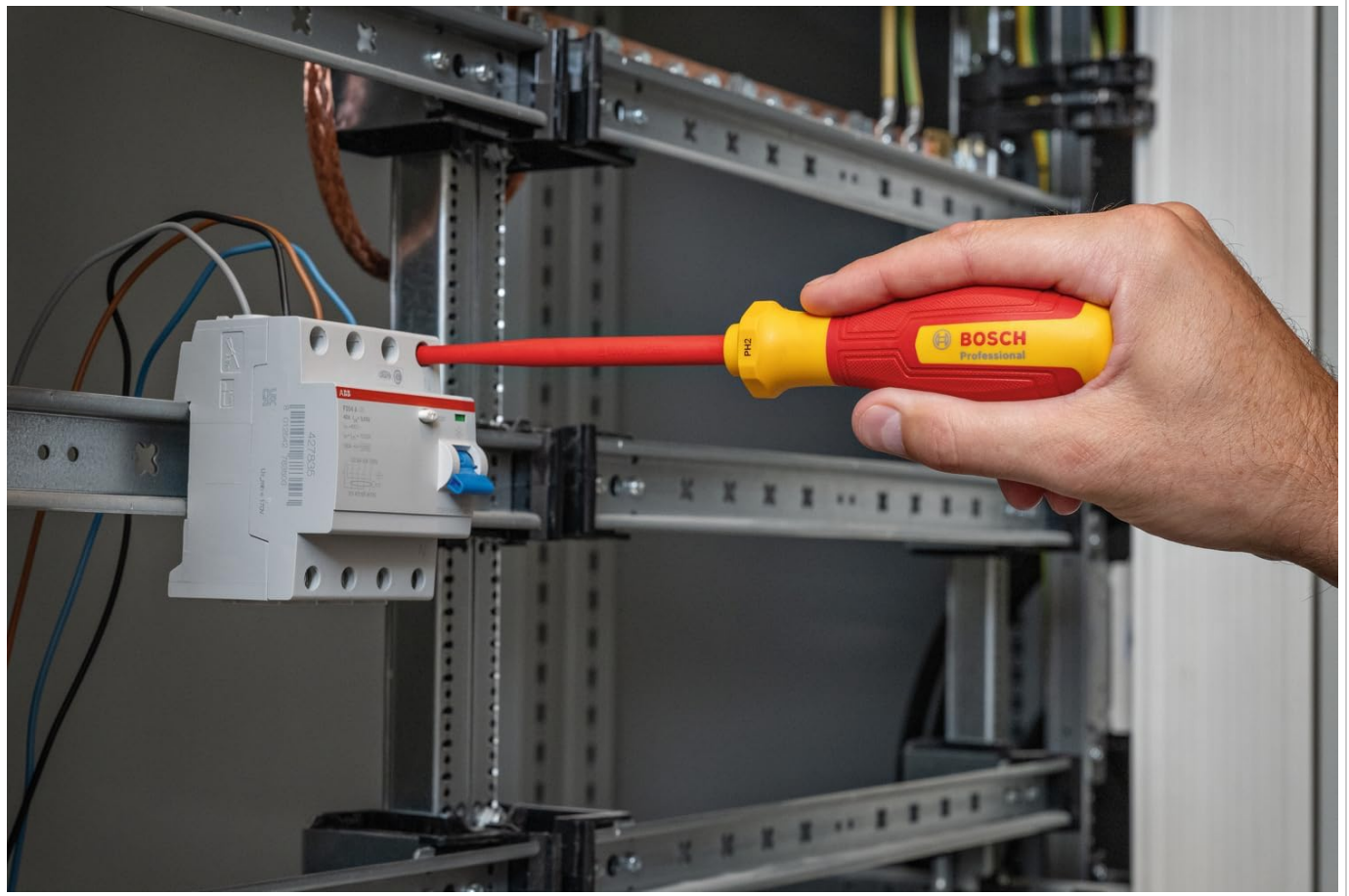
Image 5.1: Demonstrating the proper use of the VDE screwdriver in an electrical panel, emphasizing safe handling.
